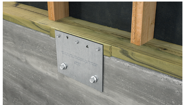
Reinforcement of the connection with the foundation
